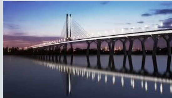
Champlain Bridge, Canada
