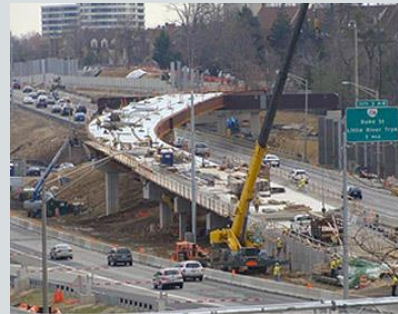
I-95 HOV/ HOT Lanes Project, Virginia
